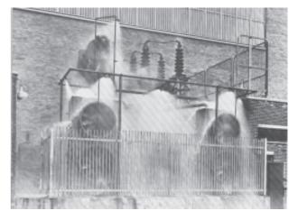
Fig-21. High Velocity Water Spray System for Transformer Fire Protection.
