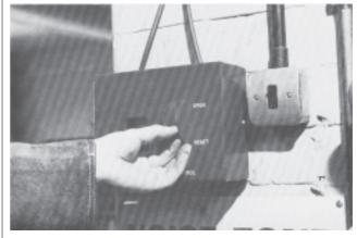
Fig. 11. Fireman's over-ride control for testing operation of fire vent installation, or for manual operation, when desired
