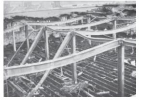
Fig. 04. Steel work affected by fire.
